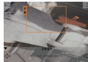
(c) 渗漏检测
